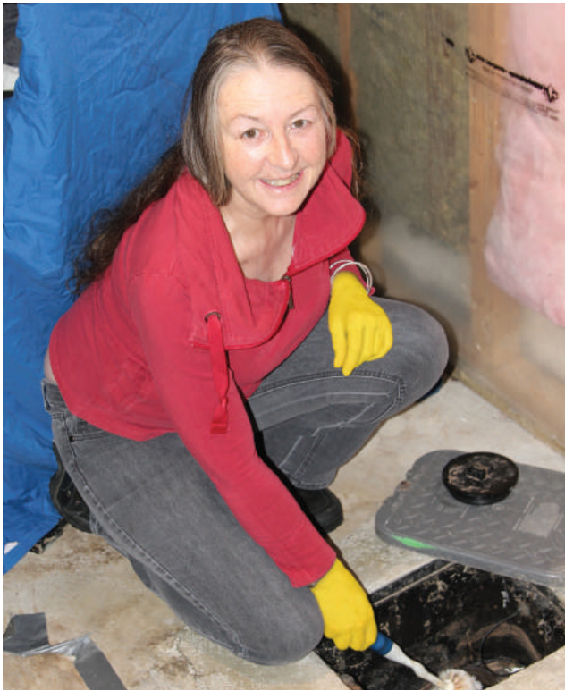
Homeowner Margaret Banks demonstrates her methods for cleaning out her backwater valve once per season to minimize risk of sewer backup. Burlington, 2017
