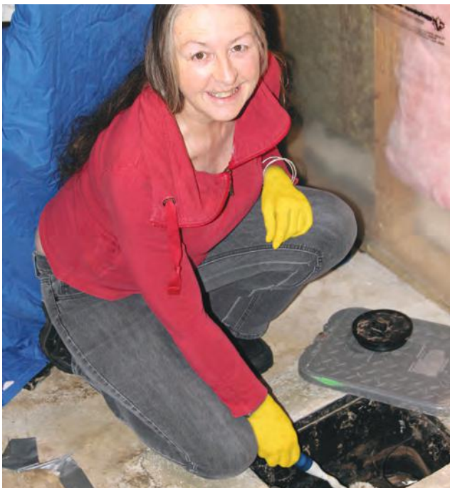
Homeowner Margaret Banks demonstrates her methods for cleaning out her backwater valve once per season to minimize risk of sewer backup. Burlington, 2017
