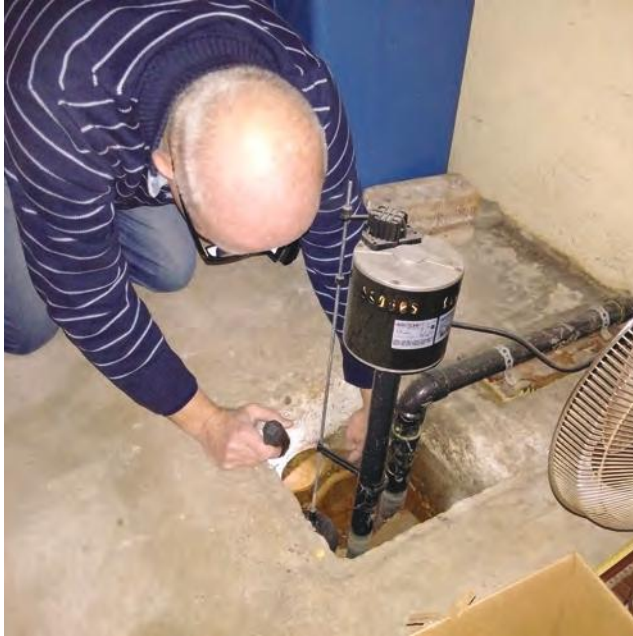
Flood Risk Assessor Trainer, Ron Bolender, demonstrates to students how to inspect a sump pit and pump. Kitchener, 2017.
