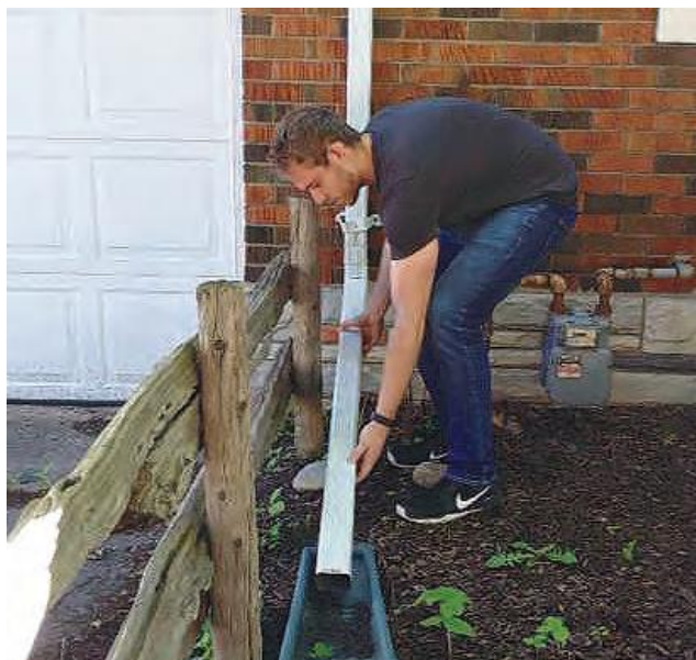
Waterloo resident Riley Davidson-Evans extends his downspouts to 2 m after his assessment. Waterloo, 2017
